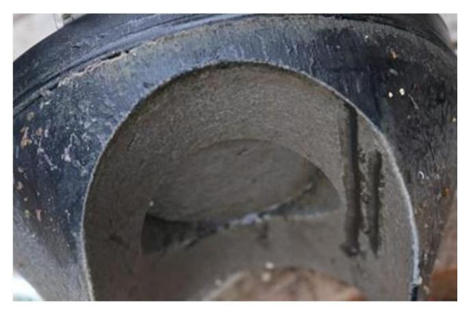
Access to the lock chamber from the top ground surface with bayonett lock with an instrument key C3 2
